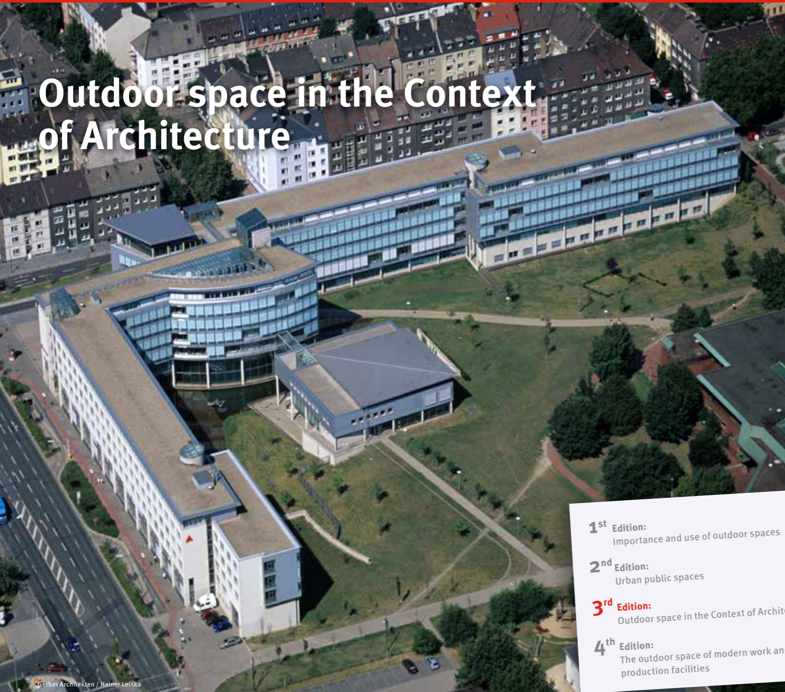
Employment Office Dortmund (GER): Two building wings run along the streets forming an angle, leaving a large part of the site shielded from the adjacent streets as a public green space. The tension between city and landscape as a basic design feature is also reflected in the façades, which are closed and clad with stones towards the outside but are filigree and transparent towards the park. (1995 Completion / 1988 Open Competition 1st Prize / Gerber Architekten)
