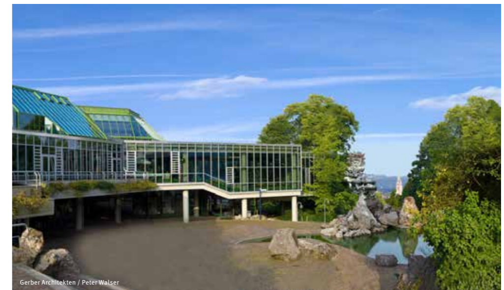
The open line of sight to Johanniskirche [St John's Church] in the centre of the city of Hagen (GER).
