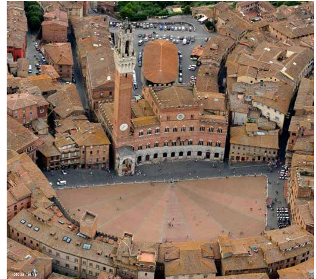
The radial structure of the square of Siena serves primarily as drainage. The water flows to the central bottom point of the shell located there.
